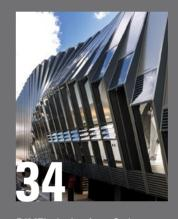
FJMT's design for a Sydney waterfront pavilion building echoes the shapes and strong-yet-light construction methods of naval vessels, with a twisting carapace of rhythmically offset composite steel panels
