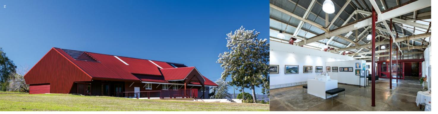
TOP LEFT: The architects have subtly modulated the depth and structure of the roof plane – made from COLORBOND® steel in Apex Apspan 700 profile and Stramit® Corrugated profile, in the colour Manor Red® – which is slimmer above the eaves and thicker above the built envelope
