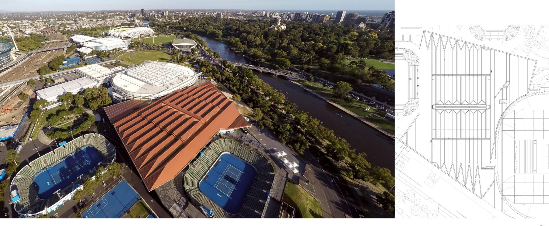
Slenderising this roof by the elimination of the usual roof tracking system introduced one of the major engineering headaches. The answer came in the form of inline wheels integrated with the roof edges to help reduce its profile from 'hamburger' to 'sandwich'. Despite being unable to track with such precision, Sheldon says they have managed to streamline the forces and overcome the tendency for excessive roof flex, potentially causing one inline wheel set to shift minutely out of alignment.
