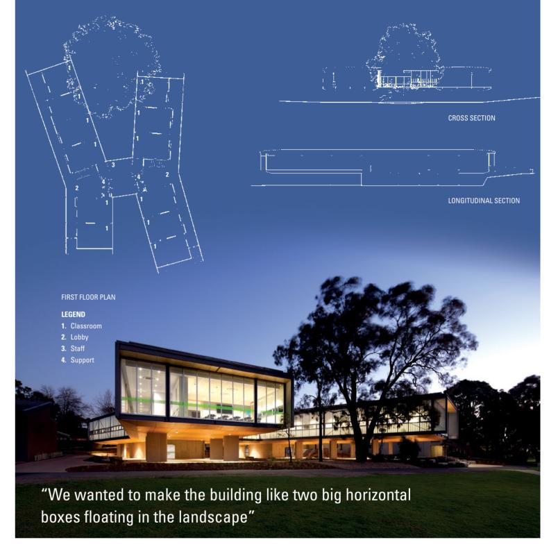
ABOVE: The structural system allows for a generous cantilever from the last column that 'floats' the pavilions 10 metres into space and creates an outdoor undercover area BELOW: The schools' grounds are cherished and the architects took this into account by extending the building's two wings around a gigantic gum tree
