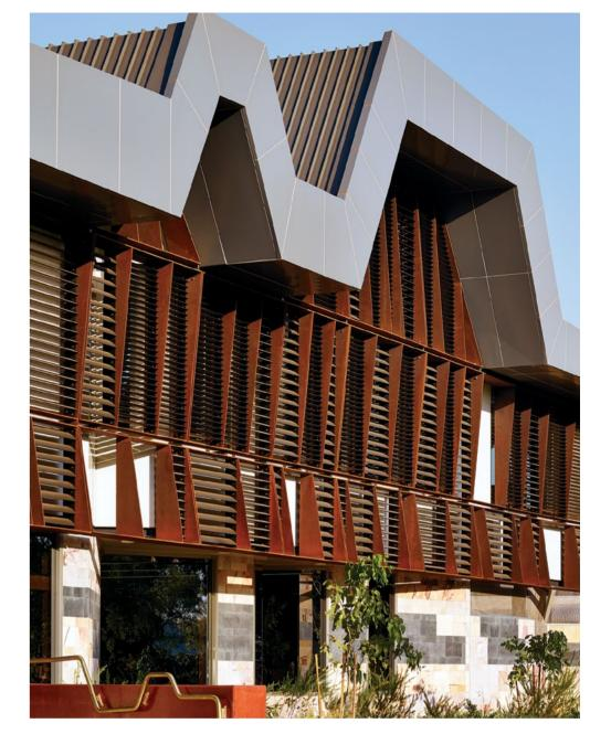
The upper levels are protected by a series of perforated screens (opposite page) and fixed metal louvres (above), all of which are mounted on BlueScope XLERPLATE® WR350 weathering steel frames. The louvres were designed to frame views - both near and far - from inside the building
