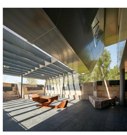
ABOVE LEFT AND RIGHT: The cave-like internal public spaces were framed using steel sections, and clad with local stone and recycled timber, to create a recognisable and familiar sensation similar to the experience of entering Hidden Valley
