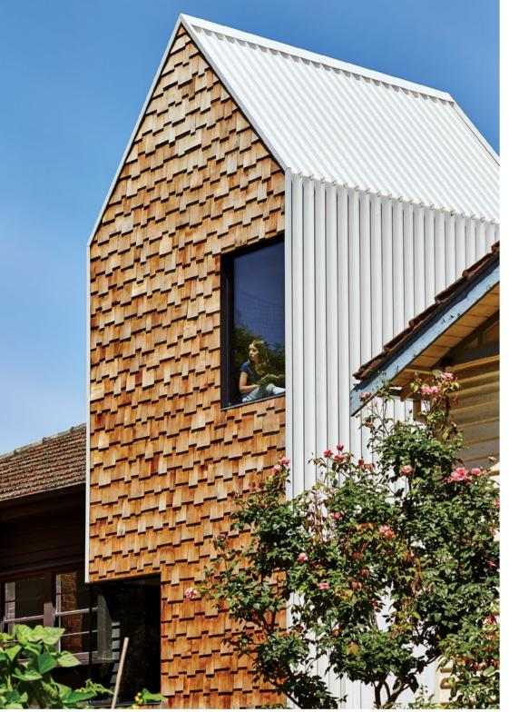
ABOVE: Twelve-metre lengths of LYSAGHT LONGLINE 305® profile made from COLORBOND® steel in the colour Surfmist® envelop each side of the tower
